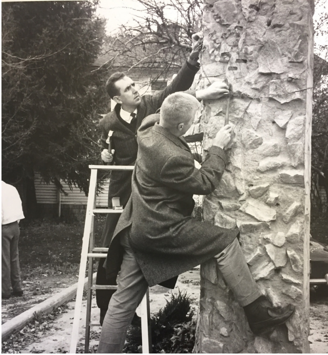
Figure 2: Cesar Pelli and John Buez during full scale mock-up of stone walls Source: Eero Saarinen Collection (MS 593). Manuscripts and Archives, Yale University Library.
