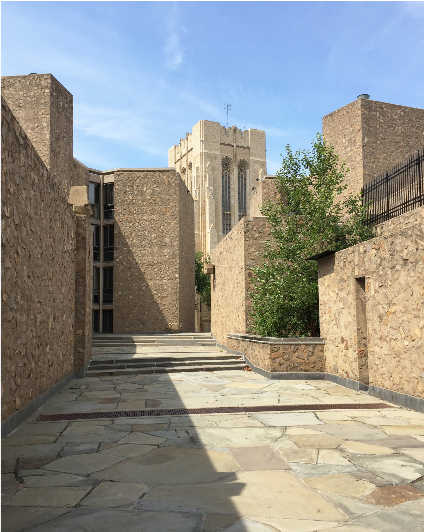
Figure 4: View through exterior passageway. Source: Benjamin Pollak © 2017
